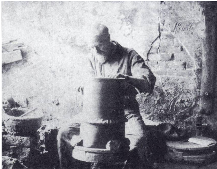
(5) Gerardus Draaisma (1860 - 1934) when making a water filter in the Groningen terracotta factory. Our family counts five generations of potters. Photo (1919): 'Fries Aardewerk'. See photos 1, 8, 10, 11, 12.
